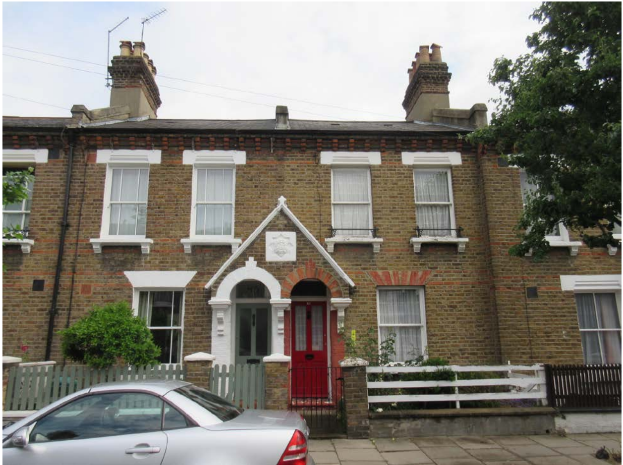
Front elevation (application site on left of photograph). (Photograph taken after removal of security box from between the first floor windows.)
